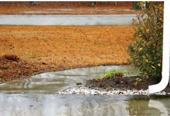
Typical placement of a downspout
