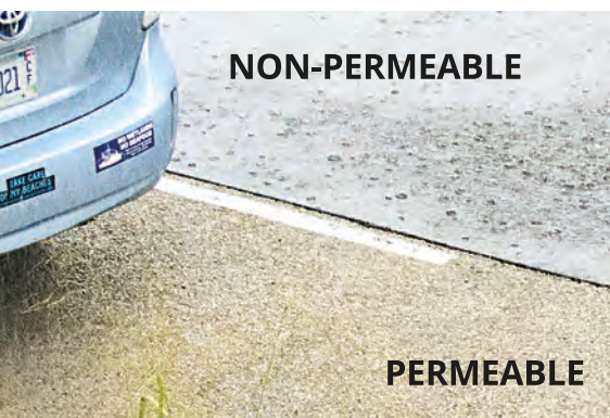
Notice how rainfall soaks into permeable pavement
