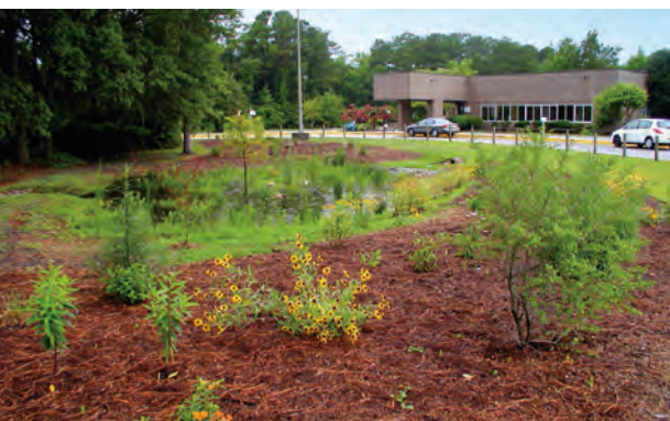
Bradley Creek Elementary School stormwater wetland
