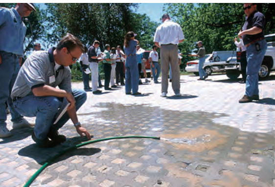
Permeable paving demonstration
